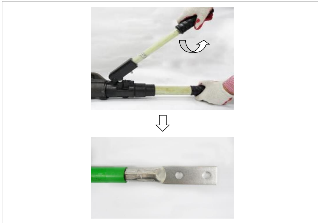
Figure 87. Fixing Pressure Terminal_Hydraulic Press (5)
