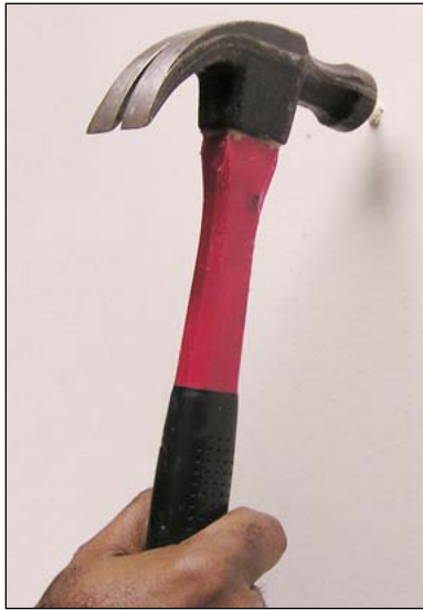
Figure 2.10 Hammering Plastic Anchors
