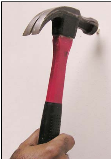
Figure 2.5 Hammering plastic anchors
