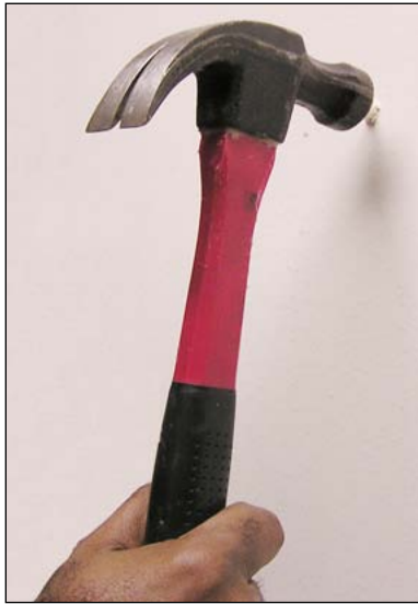
Figure 2.10 Hammering Plastic Anchors
